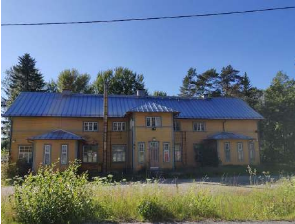
Figure 1 Accommodation building at the Oravais reception centre
