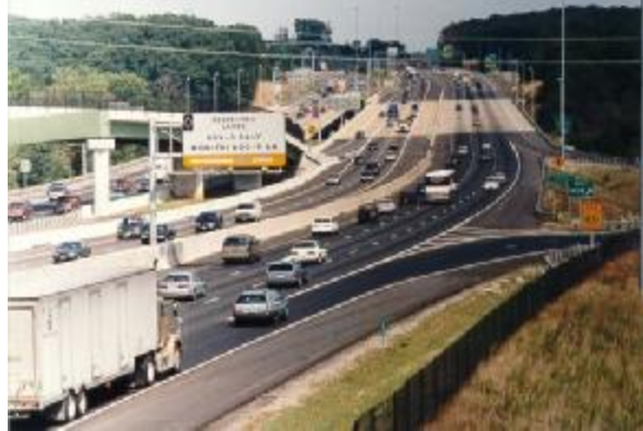
Figure 1.2. Center Two Reversible Lanes for Peak Period HOV-3 Vehicles of I-95 around Washington D.C. Area (roadtothefuture.com)
