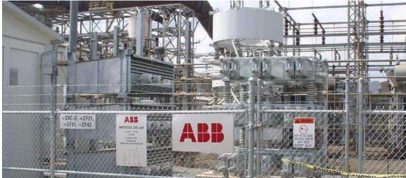
(a) 64 Mvar static VAR compensator
