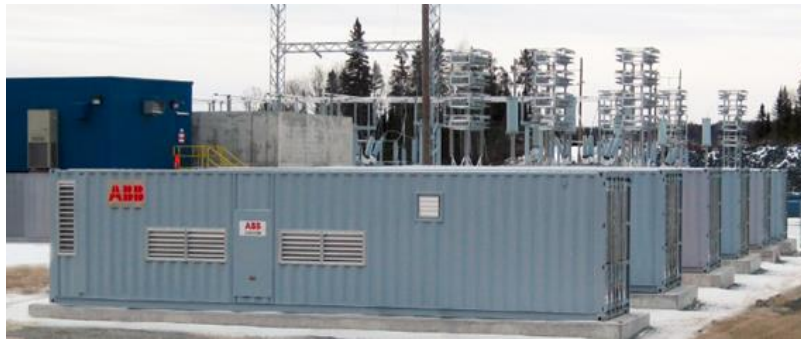
(b) Six 4.5 Mvar static synchronous compensator
