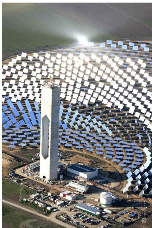
Fig. 1. Abengoa PS20: a 20Mw solar power tower
