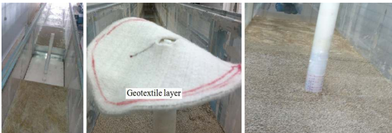
Fig. 1 Pier model installation in the flume
