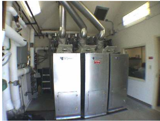
Figure 12: Inside of the Test Facility
