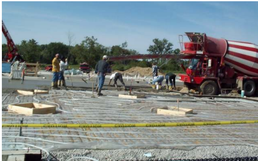
Figure 14: Hydronic Radiant Floor Heating System Installation
