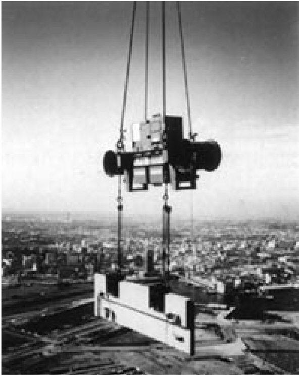
Fig. 7. Actively Controlled Crane used during Construction of the Yokohama Landmark Tower
