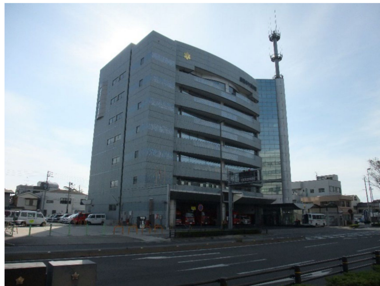
Figure 4. Toyohashi Fire Station Building.
