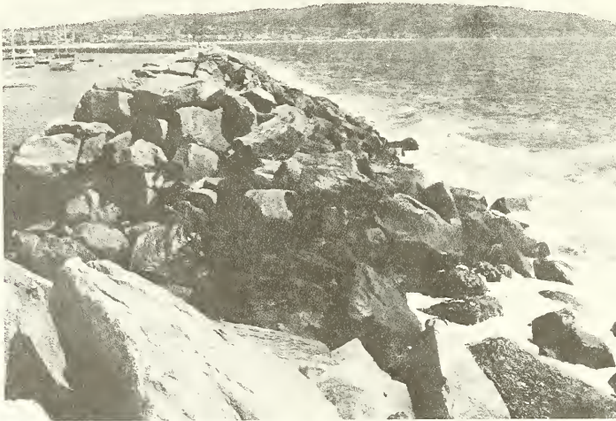
Figure 1. A rubble-mound breakwater protecting a boat harbor
