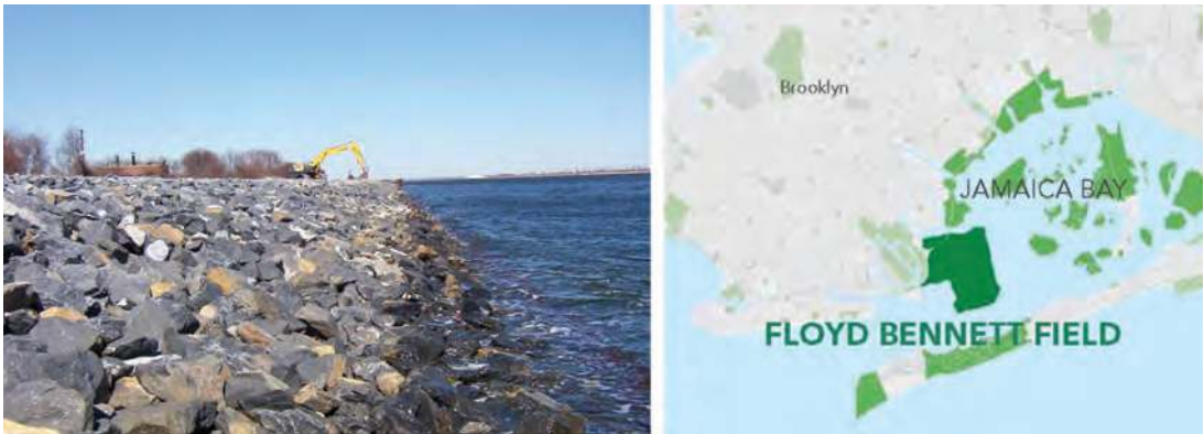
Figure 3.3. New graded bank protected by stones replaced the old steel bulkhead at Floyd Bennett Field, Jamaica Bay, Brooklyn (source: Ap Construction, 2012).
