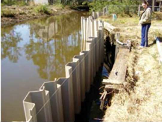
Figure 3.2. Example of vinyl bulkheads (adapted from Ecobuilders, 2012).
