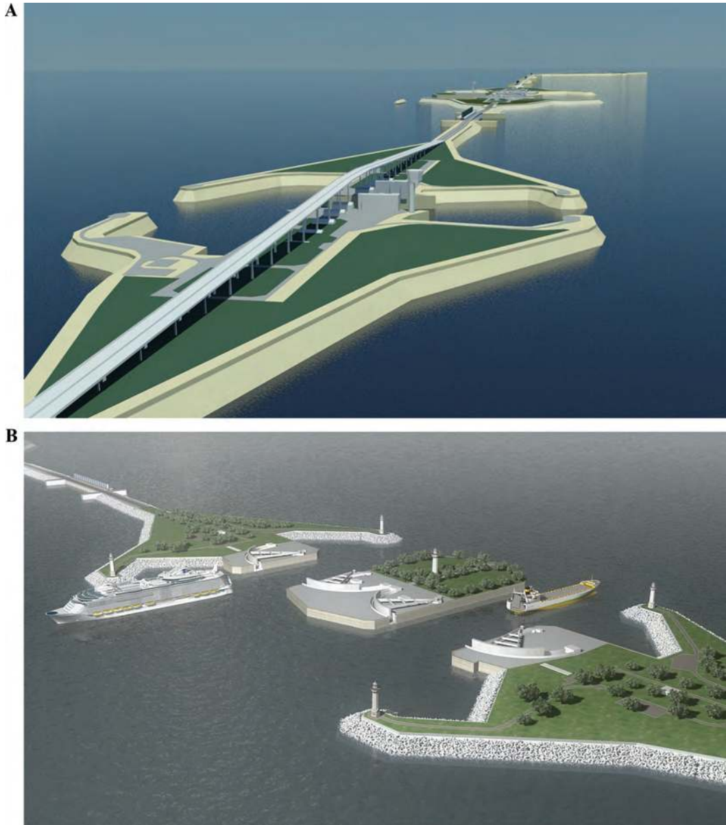
Figure 4.11. Causeway over sluice and barrier system ( Top ); navigable floating sector gates at the Ambrose channel ( bottom ) (source: CH2 m).
