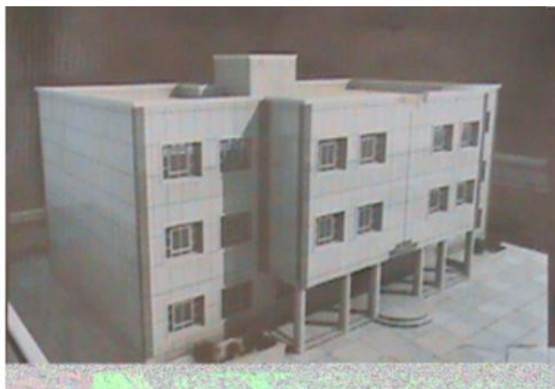
Fig.5 The shape of school building.
