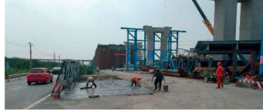
FIGURE 13: Ground enhancement for crane settlement.
