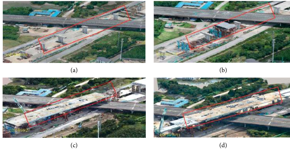
FIGURE 16: 3D models reconstructed from UAV for visualization and off-site monitoring. (a) May 16, 2018, (b) July 10, 2018, (c) Sep. 27, 2018, and (d) Oct. 11, 2018.
