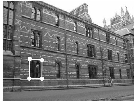
Figure 1: An image with significant perspective distortion. Four points, corresponding to the corners of the rectangular window, fully define a rectification homography for the plane of the building facade.
