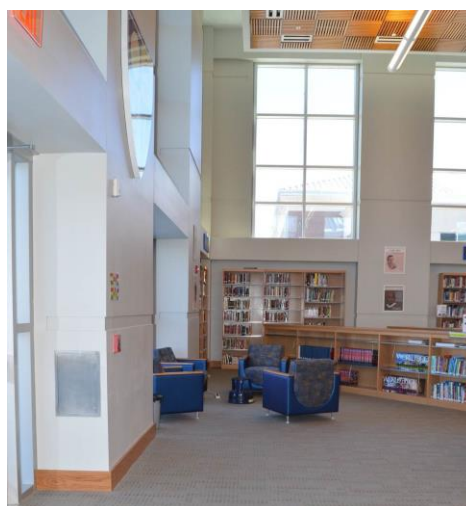
Figure 5.1.1 G: Site A – View of the East wall of Library
