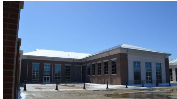
Figure 5.1B: Site A – Back View of Main Building (Court Yard)
