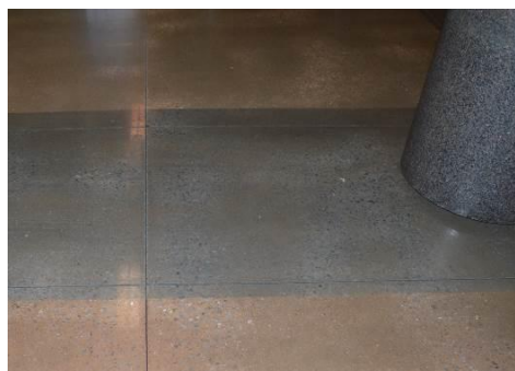
Figure 5.1.1E: Site A – View of Polished Concrete Floor
