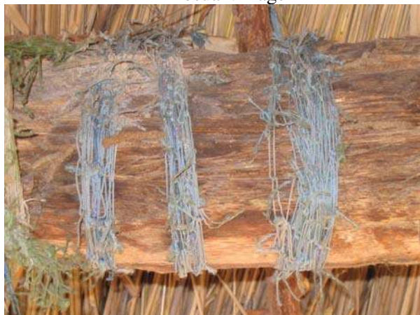
Figure 3.28 Old net used for roof construction in Akosua Village
