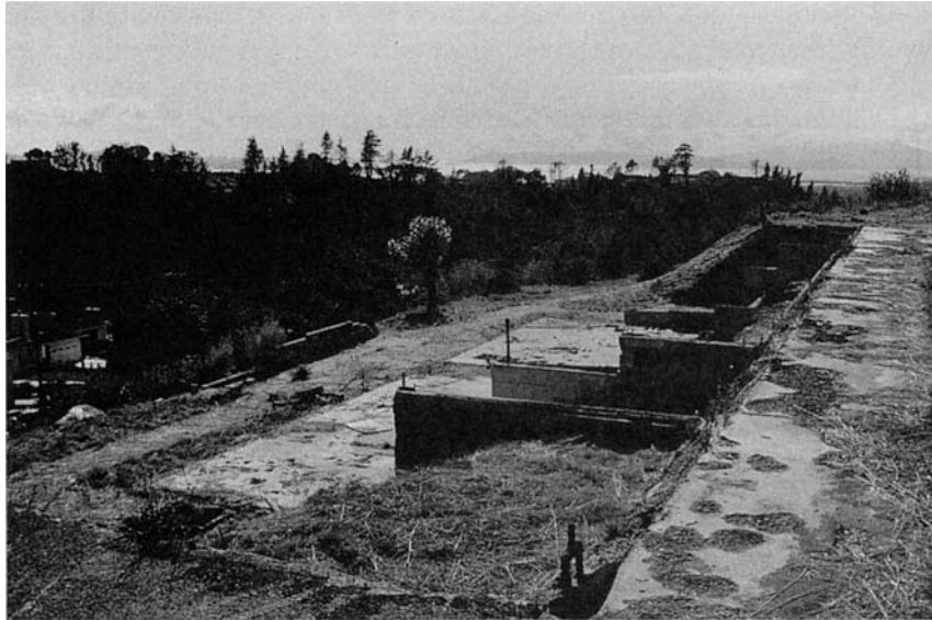
Photo 10.1 Concrete foundations were all that remained of hundreds of homes burned in the Oakland firestorm
