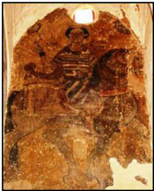
Figure 4. Detachments of parts of plaster.
