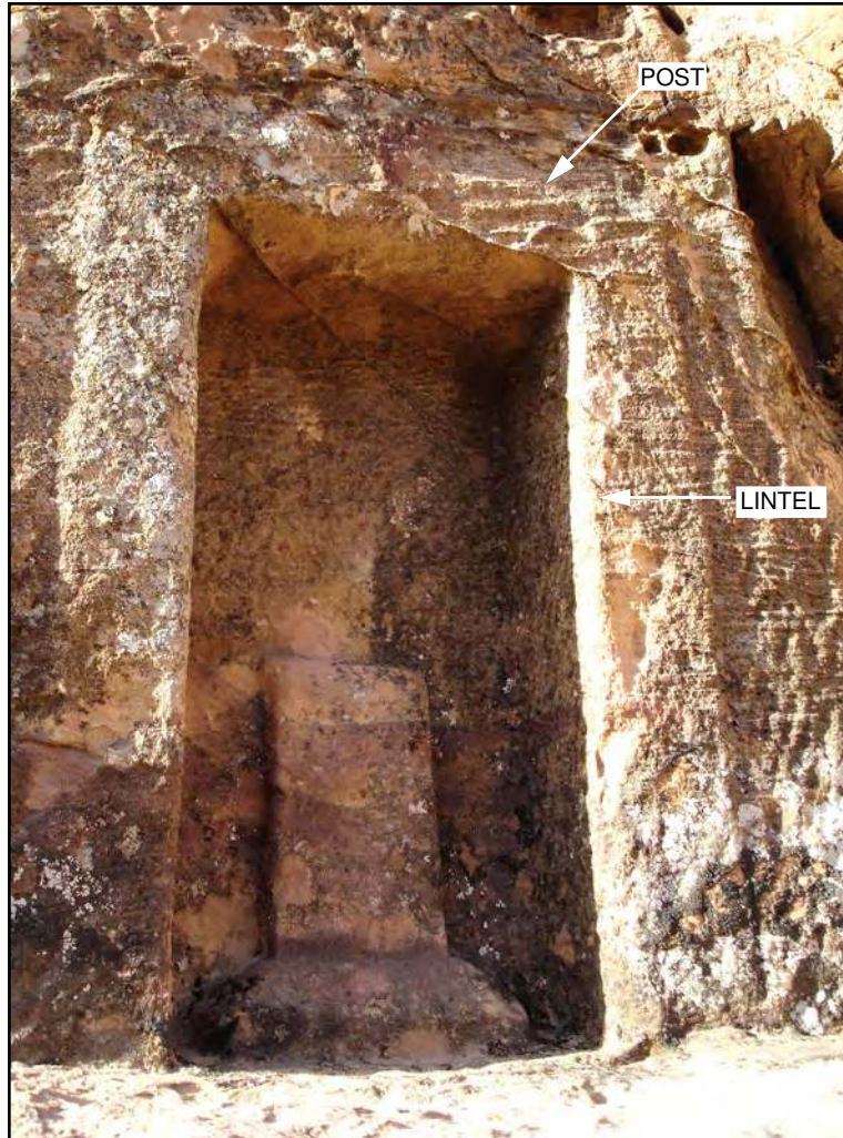
Figure 5.39. Example of a Type I Facade in Area C (Niche 19).
