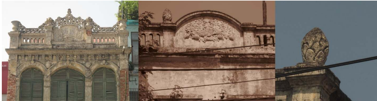
Figure 1: Pictures of old houses in Hanoi showing French architecture and Confucian, Taoist and Buddhist symbols were added together.
