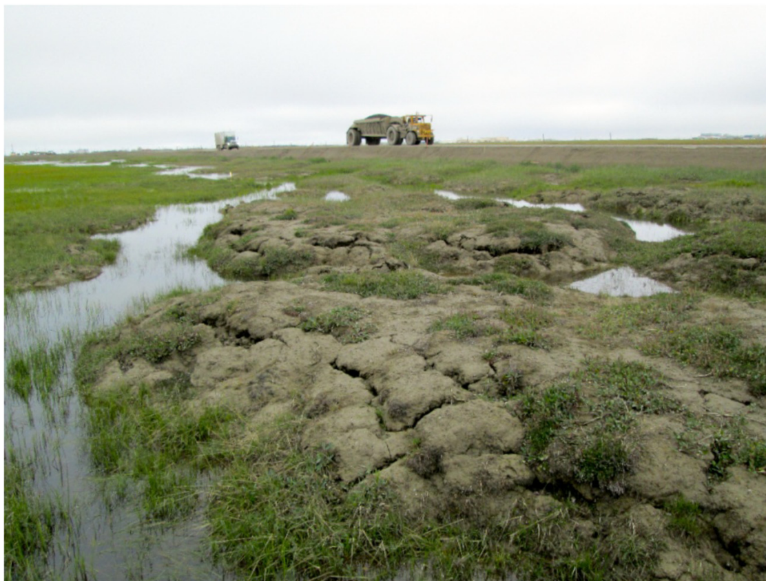
Fig. 1. Roadside area through a network of ice-wedge polygons, Prudhoe Bay Oilfield, Alaska. Roadside flooding, road dust, and other impacts have caused subsidence of the ice-wedges and erosion of the polygon centers. Here, low-centered polygons have been converted to high-centered polygons, altering ecosystems in a wide swath of tundra adjacent to the road.
