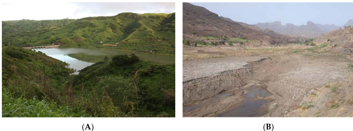
Figure 6. Poilão dam in São Lourenço dos Órgãos at the Santiago Island (A) Rainy season; (B) Dry season). Photos taken by the authors (MMR and APE).
