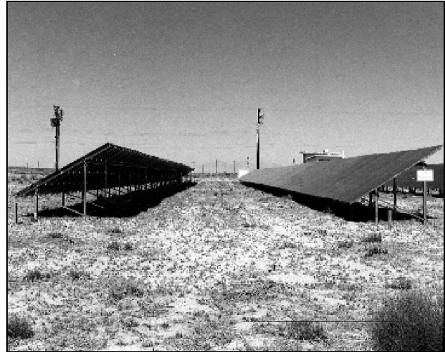
Fig. 6: A 25-kW thin-film CdTe array deployed at Edwards Air Force Base, California.
