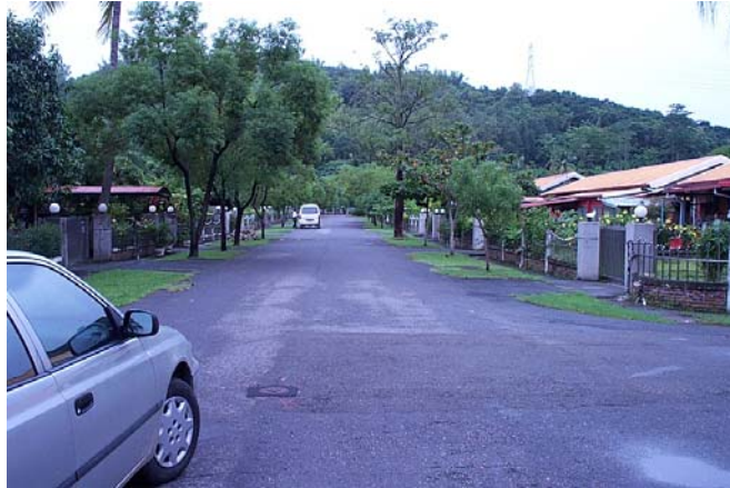
Figure 2. Photo P-1 showed the single-story residential building in the east side of Wufeng Site A (by D. Chu, 2001)
