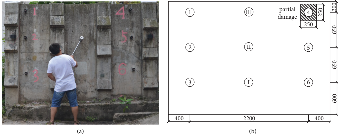
FIGURE 1: Vibration tests on the pile plate wind-break wall. (a) Loading impulse excitation. (b) Position of the measurement points and partial damage.
