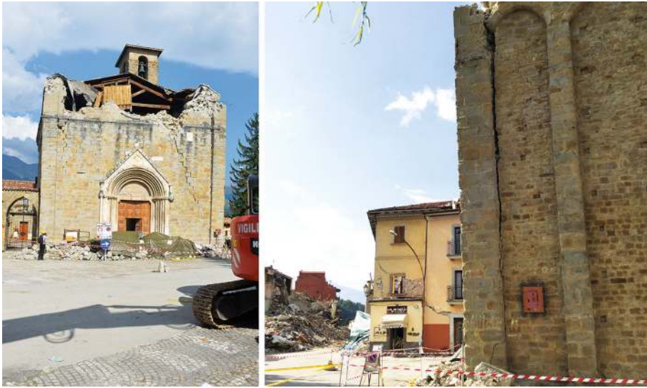
Fig. 25 Church of S. Agostino: damage level D4, collapse of tympanum (M6) and in-plane cracking of façade (left); overturning of façade (M3, right), ev1 vulnerability factor
