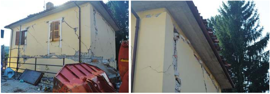
Fig. 22 Residential masonry building: D3 damage level, in-plane cracking shear mechanism (M2), poor masonry vulnerability factor (ev4)
