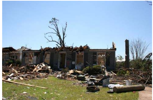
Figure 4.13 Single family dwelling with DOD of 5 to 6.
