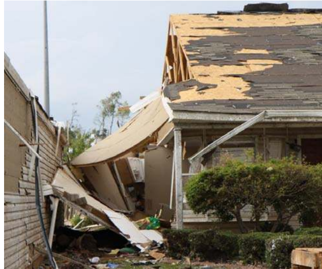
Figure 4.3: Exterior wall and gable roof end pulled out as a result of high leeward winds
