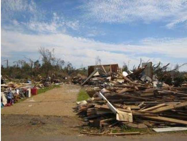
Figure 5.12 Most walls collapsed
