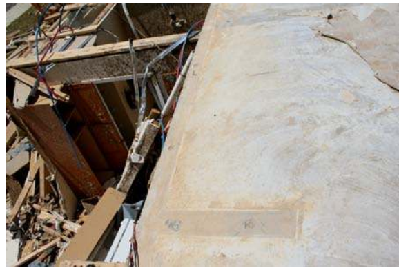
Figure 4.10 Slab swept clean with cut nails at edge
