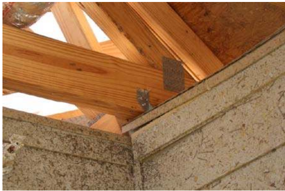
Figure 4.9 Photograph of installed hurricane clip
