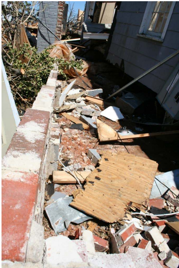
Figure 4.4 House lifted off its foundation. Chimney shown to the right approximately 5ft over.
