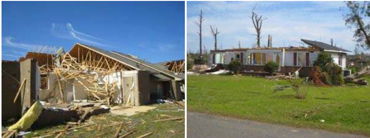
Figure 5.10 Large sections of roof removed
