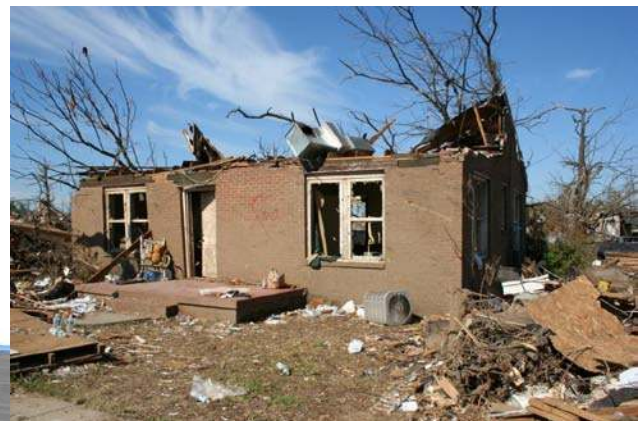
Figure 4.1: loss of roof assembly
