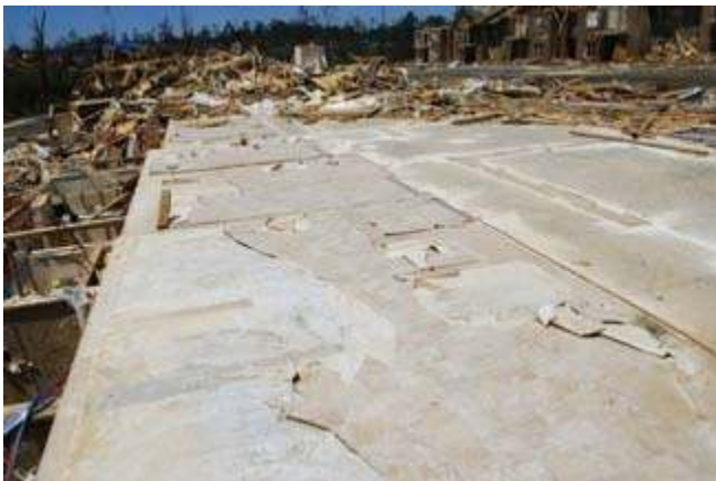
Figure 5.13 Slab swept clean in newer 2010 construction
