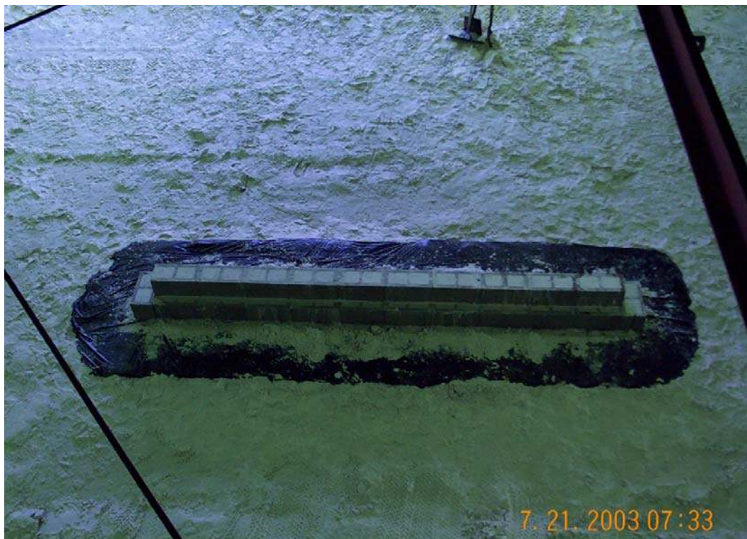
Figure 29. Third layer concrete block breakwater core.
