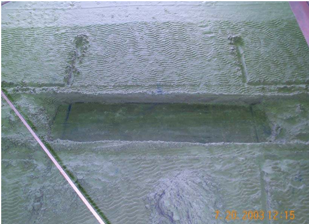
Figure 26. Excavated sand beach for breakwater construction.
