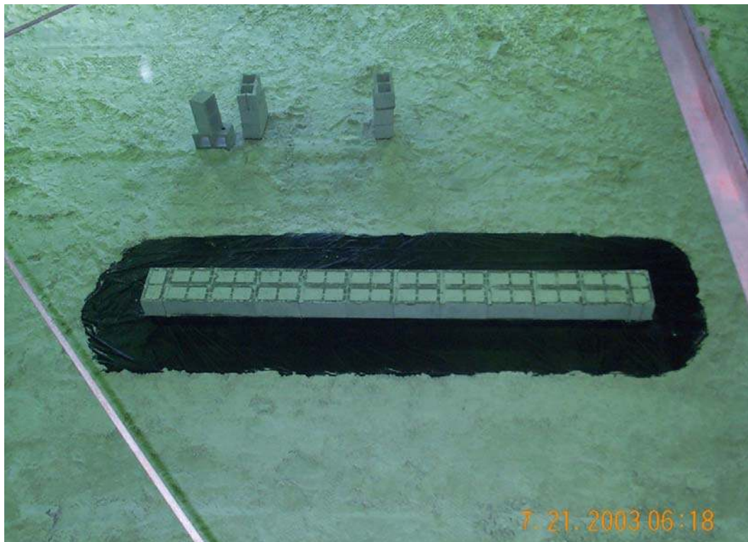
Figure 28. Filter cloth covering foundation and second layer concrete block core.
