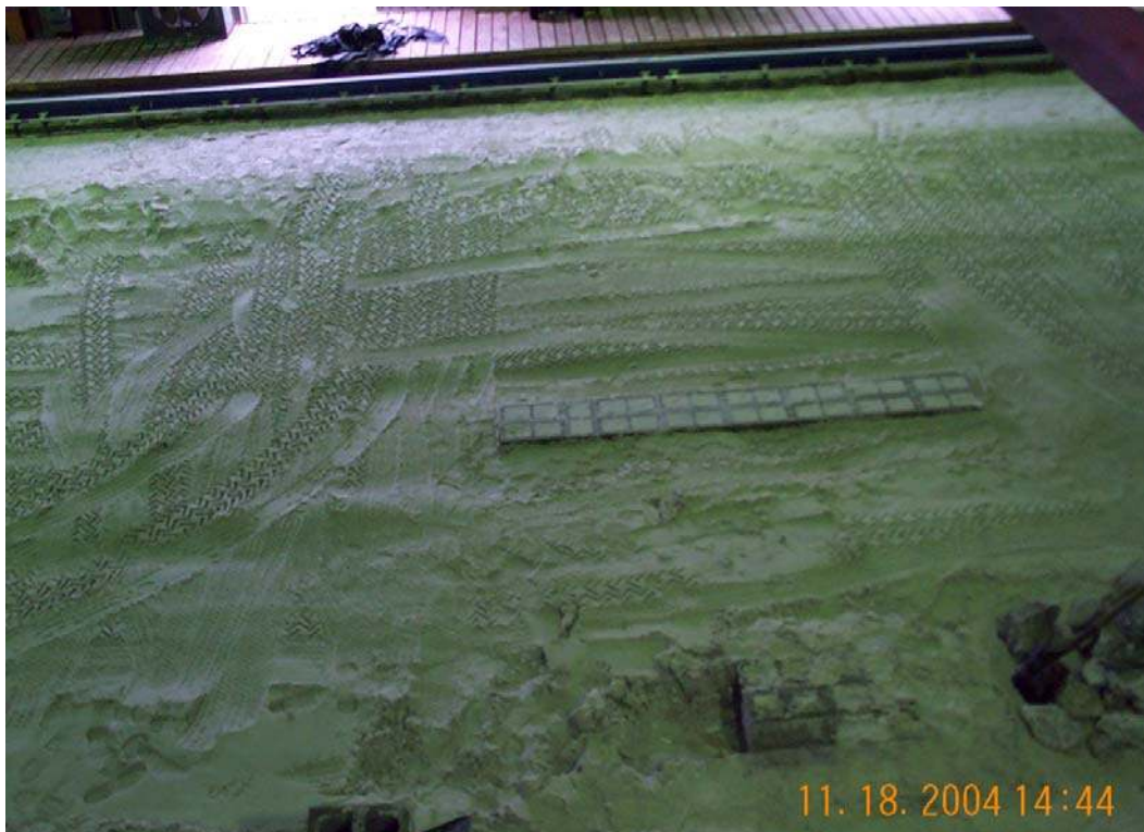
Figure 142. Breakwater foundation and core.
