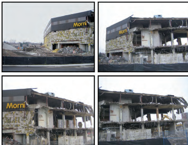
Figure 6 Morningside Mall demolition (source: courtesy of East Scarborough Storefront)
