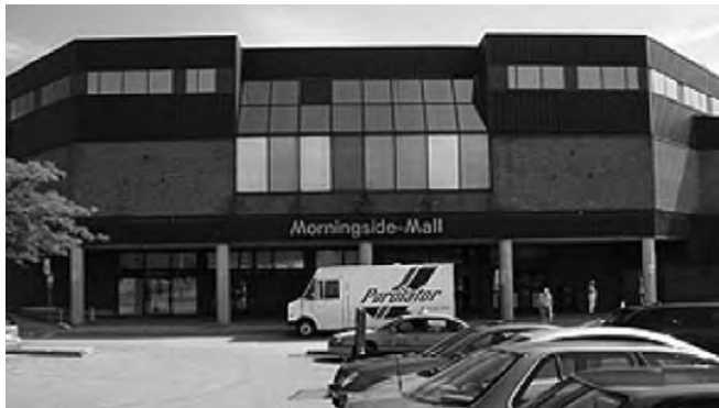
Figure 5 Morningside Mall prior to demolition (source: Author’s photo, 2005)
