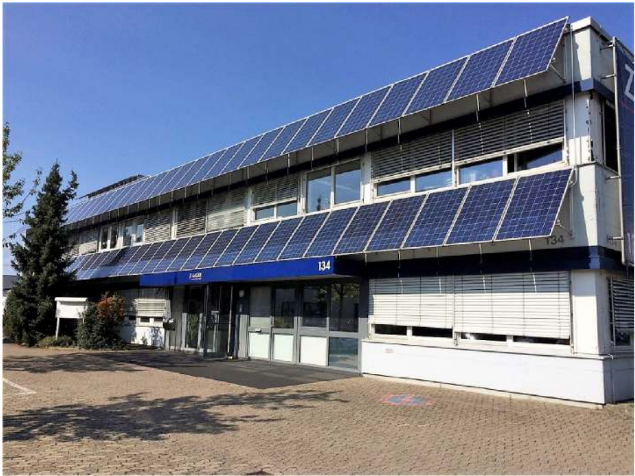
Fig. 1 Building integrated solar panels at the Intelligent Solutions in Light Offices in Vauban, Germany, September 2018. Source: Authors
