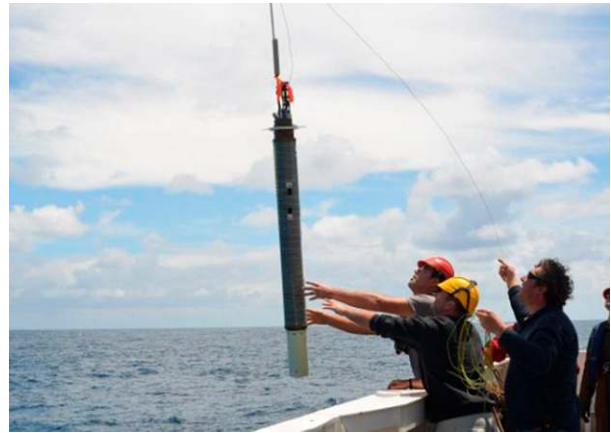
FIG. 11. Deep-Arvor deployment during Geovide cruise, May 2014. The float is suspended by its damping collar with a handling rope and then launched at the sea surface by means of a trigger snap shackle.
