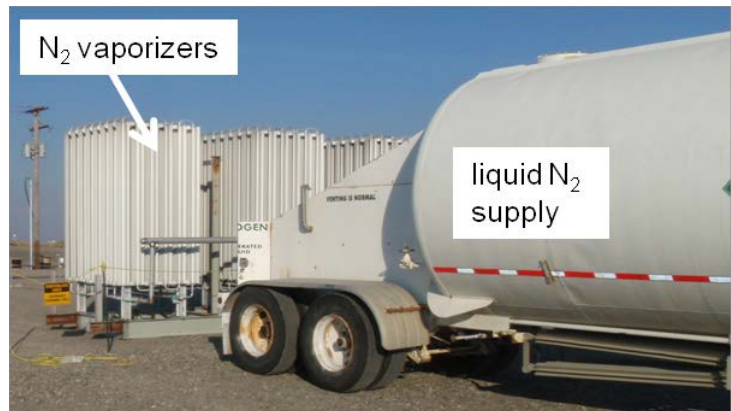
Liquid Nitrogen Supply to Produce Nitrogen Gas for Injection
