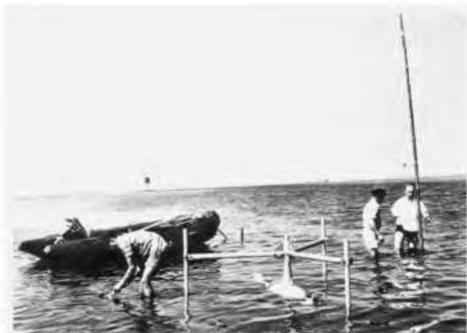
Fig. 10 Recording current meter for use in tidal flats
