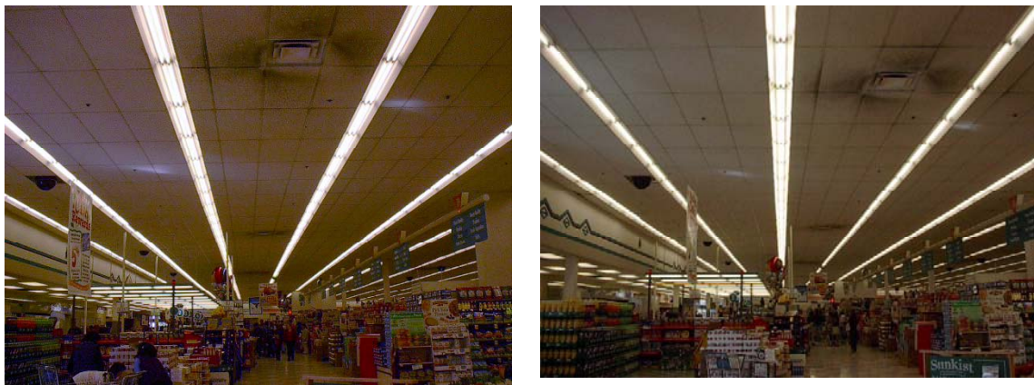
Figure 6: Overhead lighting at normal (left) and in load shed mode (right). In load shed mode, about 50% of the rows of lamps are switched off.
