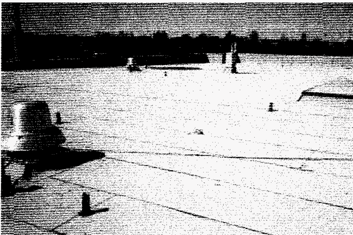
Figure 2.2 Rooftop of the Kaiser Permanente Medical Office Building in Davis, California, light gray capsheet with solar reflectance of 0.24.
