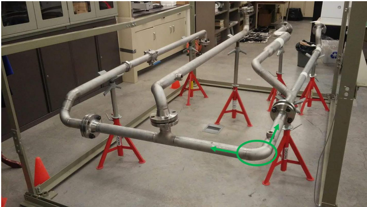
Figure 55: Photography of the steel pipe assembly located in the UW lab. The green oval surrounds the elbow. Each green arrow is pointing at an area of the assembly.
