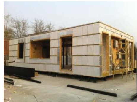
FIGURE 5: Building's exterior wall with HIPs employed during the building process (source: authors' own data).
