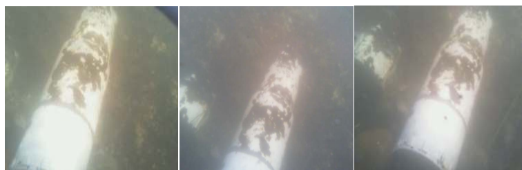
Figure 23. Images of connections between PVC pipes placed underwater.
