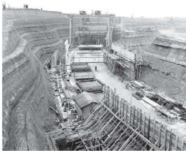
Fig.12: The excavation of the ISR tunnel
