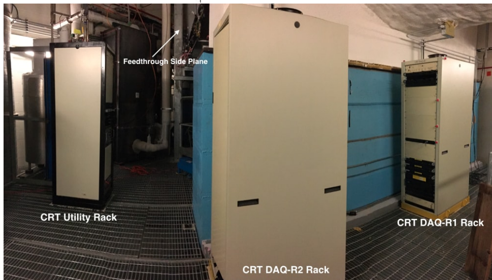
Figure 12: CRT racks in the LArTF pit. Three racks are located in a free area at the downstream beam end under the cryostat and next to the feedthrough side plane.
