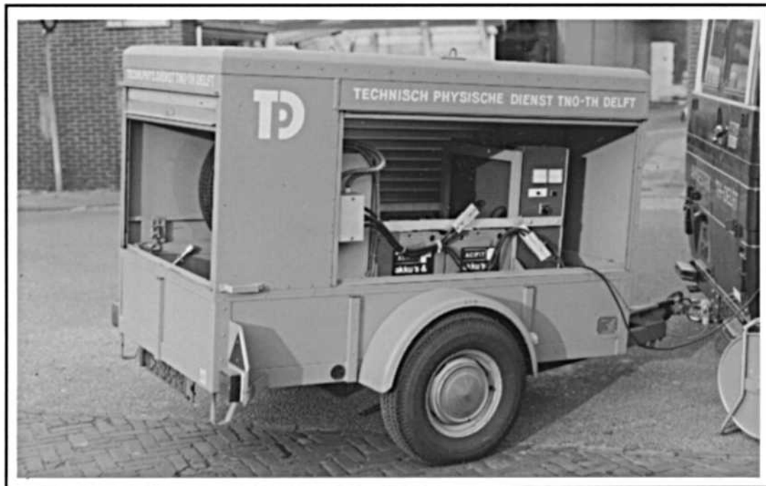
Figure 4.6: The battery-operated 220 V/ 50 Hz power supply of the TPD, mounted on a trailer.
