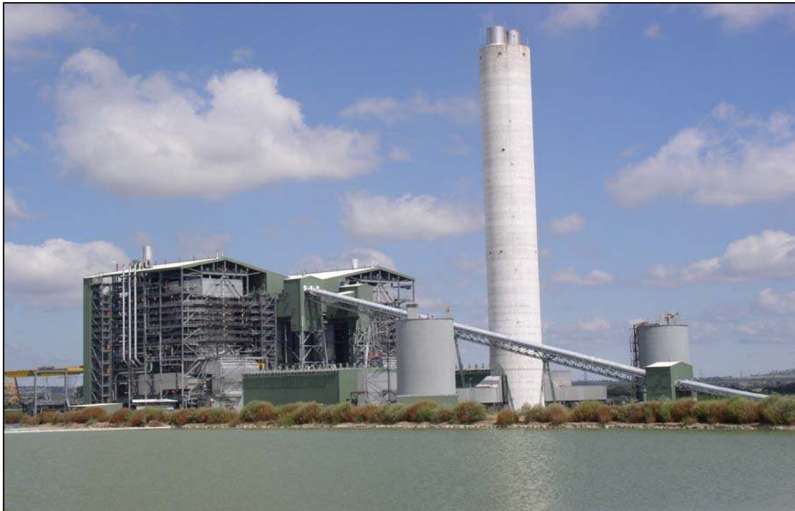
Figure 4.1: Millmerran Power Station
