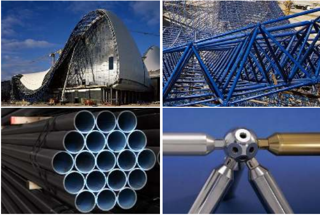
Fig. 2. The Heydar Aliyev Cultural Center (top-left) in Baku, Azerbaijan was designed by Zaha Hadid. The supporting space structure (top-right) underlying the freeform surface was constructed by MERO-TSK using circular hollow section tubular beams (bottom-left) and the KK-Ball Node System (bottom-right).
