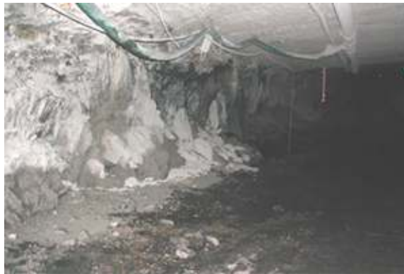
Figure 6-11 Small rib fractures at 1000 ft deep
