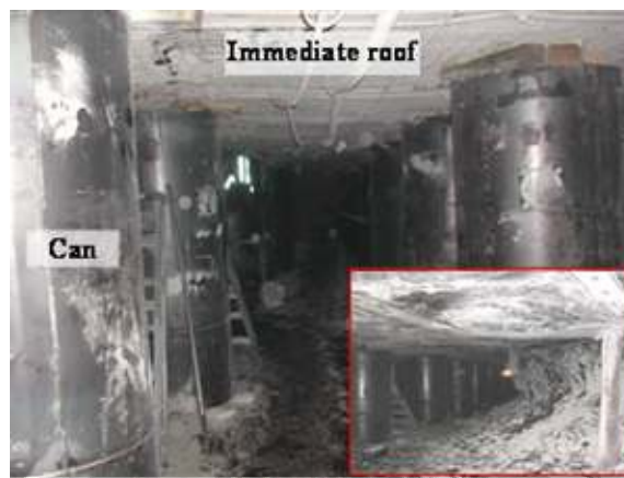
Figure 6-7 Cans installed in the tailgate
