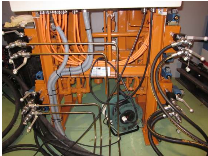
Figure 6. Valve blocks installed.
