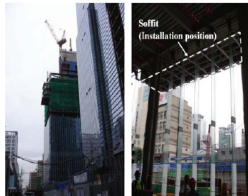
Figure 1 Construction Site and Installation Position
