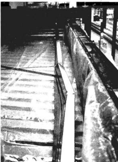
Figure 8: Purlin test Failure mode under wind suction load
