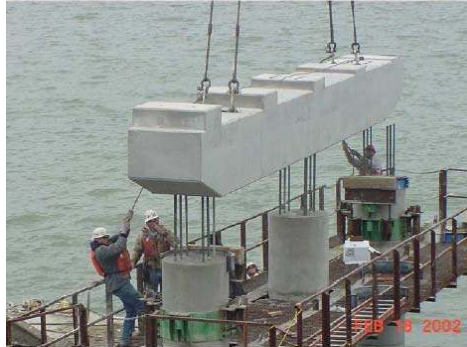
Figure 4: Precast Bent-Cap Installed on Site (Texas DOT)
