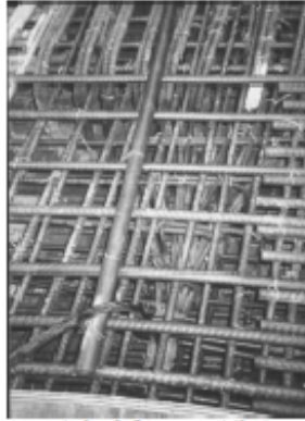
Figure 10: Congested Reinforcements
