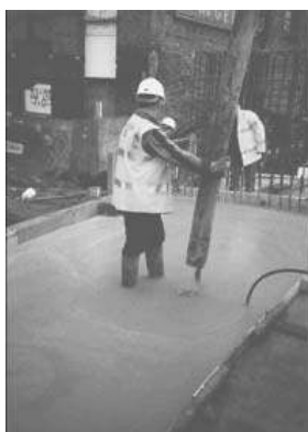
Figure 9: Self-Compacting Concrete being cast
