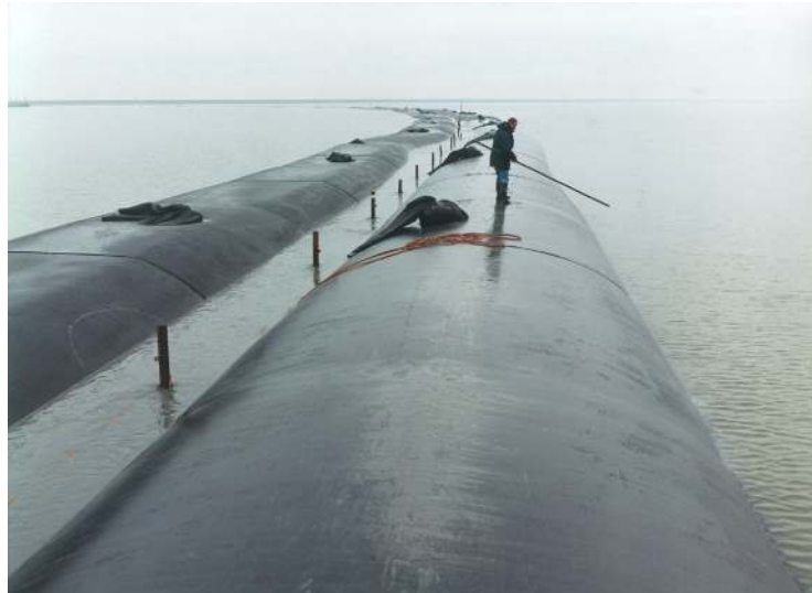
Figure 16. Example of construction of breakwater using geotubes
