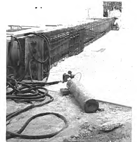
Fig. 19. Forms with inflatable rubber voids.
