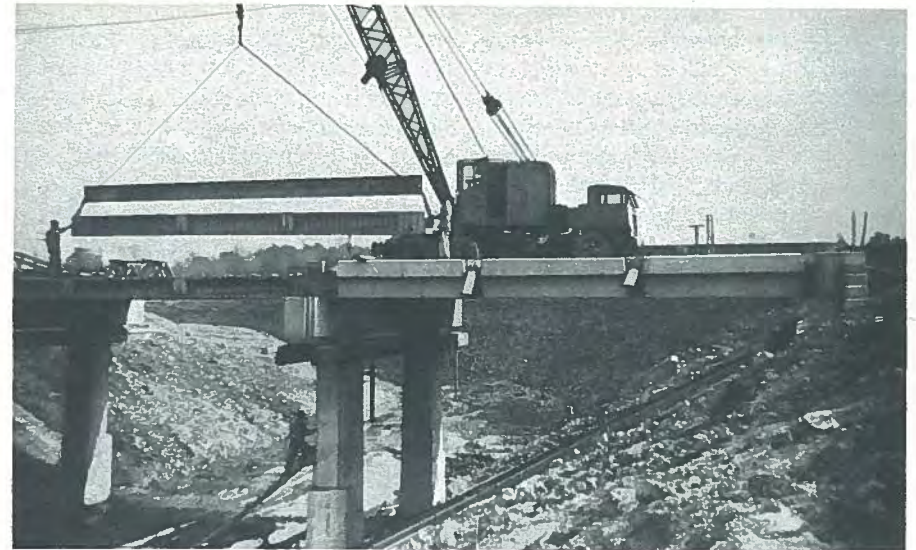
Fig. 16a (top). Erection of typical block-beam in Michigan.
