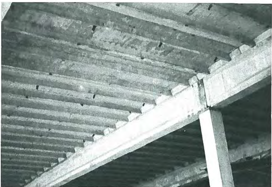
Fig. 10. A 6-ft (1.83 m) wide double-tee was developed from existing channel slab designs to allow larger spans between beams in the cold storage warehouse for Beatrice Foods.
