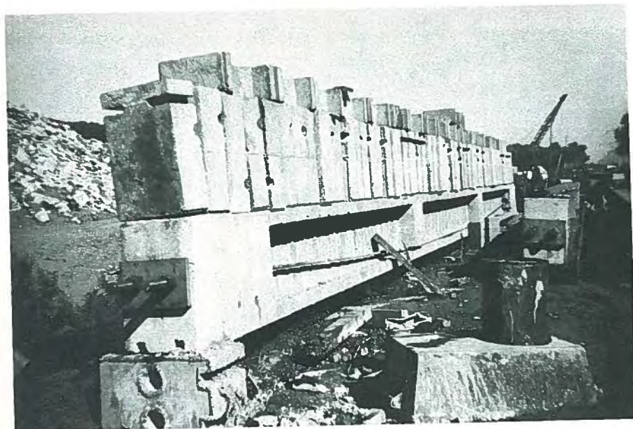
Fig. 15. Testing of Michigan block-beam with 1.5 live load.
