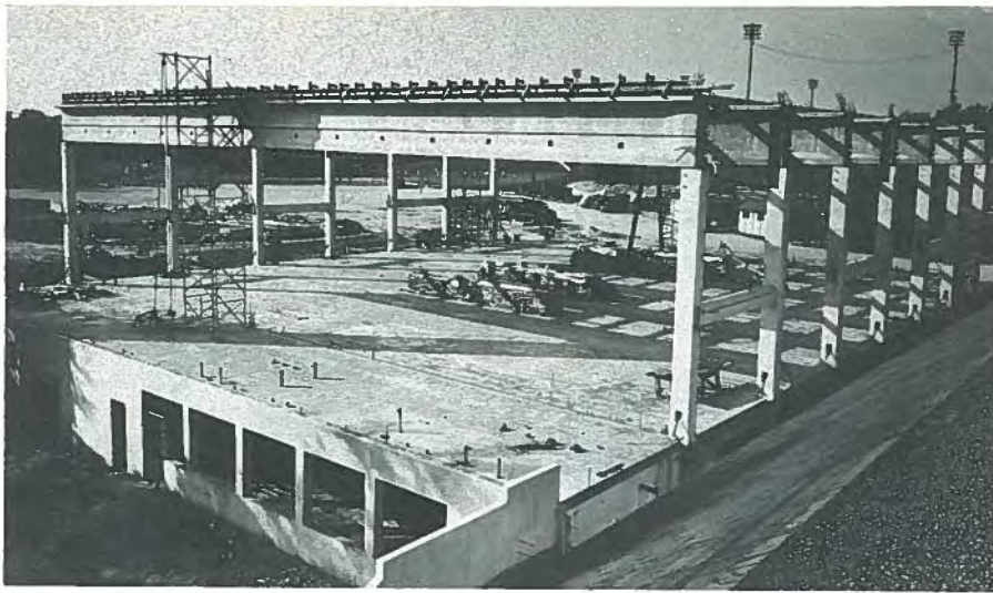
Fig. 41. All prestressed girders in place for Greensboro, North Carolina, Senior High School gymnasium.
