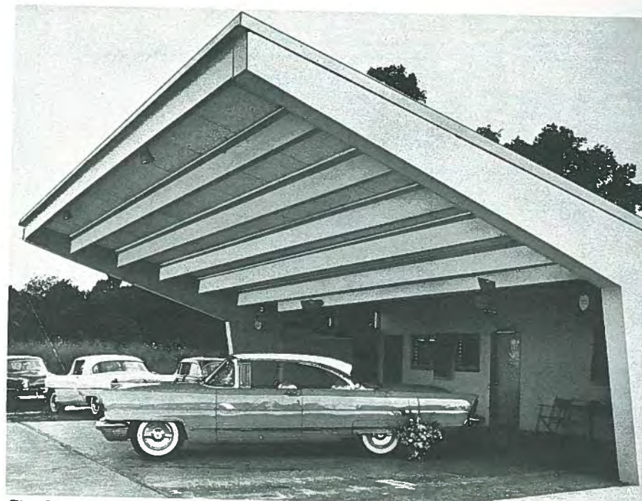
Fig. 20. Canopy using prestressed tee-joists and tectum roof deck. At one time in the mid-fifties this roofing system was quite popular in Florida but soon gave way to the double-tee.
