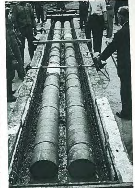
Fig. 20. Girder is about half cast, showing paper tubes used to form voids in the concrete.
