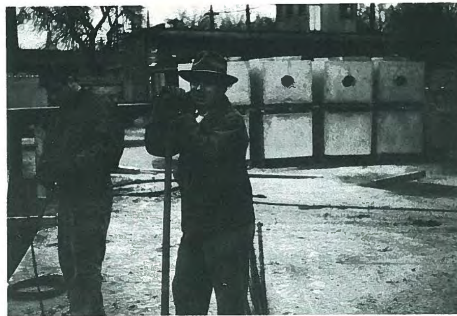
Fig. 5. Jack Perlmutter (right) and Michael Altenberg were among many men who worked day and night on Prestressed Concrete of Colorado's first pretensioning bed. The original 50-ft (15.2 m) bed was the beginning of the remarkable growth of prestressed concrete fabrication in Colorado.
