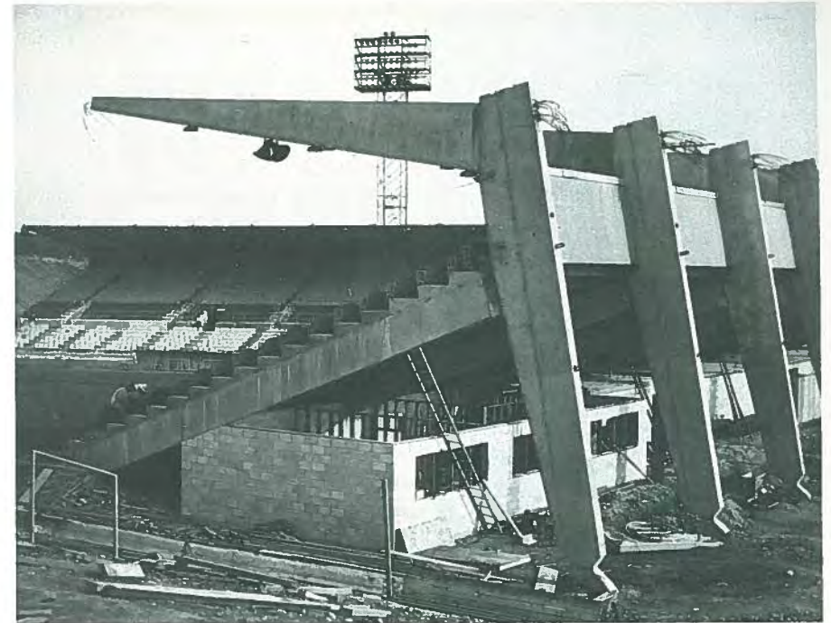
Fig. 68. Cheney Stadium in Tacoma, completed in 3½ months, did much to publicize the usefulness of prestressed concrete.
