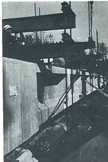
Fig. 7. Looking east, showing loading arrangement on Walnut Lane test girder. Steel ingots are in foreground.
