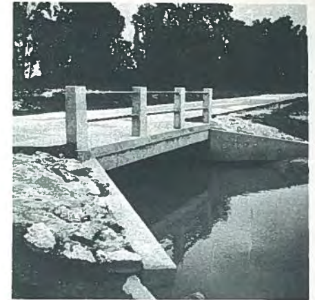
Fig. 14. Application of 14-in. (356 mm) double-tee for short-span farm-to-market bridge. Several hundreds of these bridges have been in use for over 20 years with excellent performance.
