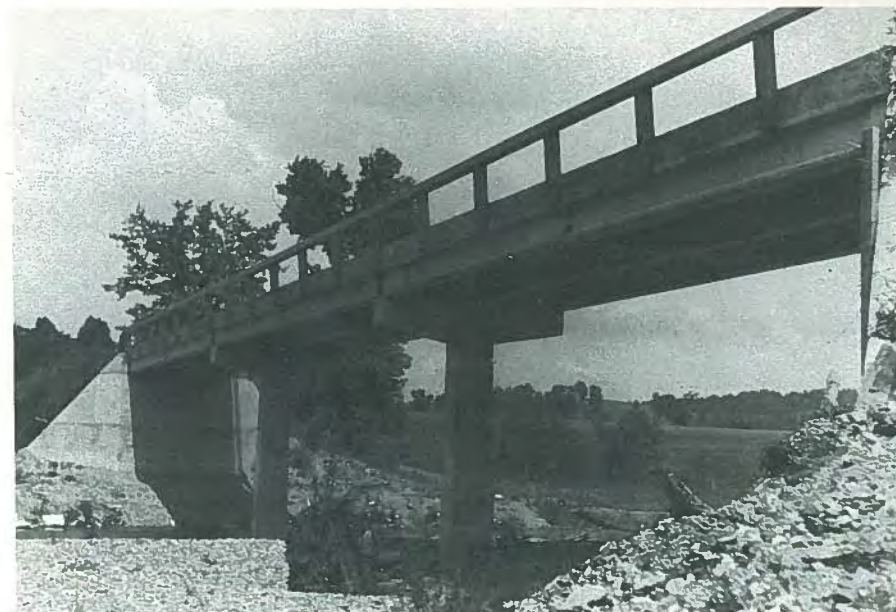
Fig. 18. Cheatham County Bridge of three 50-ft (15.3 m) spans made continuous by reinforcing in composite pour over supports. Pier caps are precast. Built in 1955.
