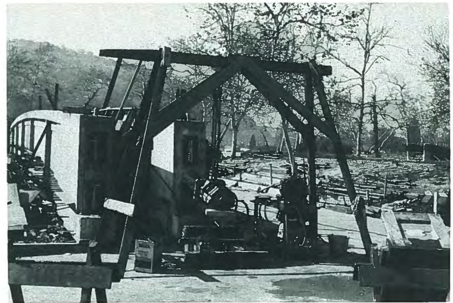
Fig. 10. Stressing the Arroyo Seco girders.
