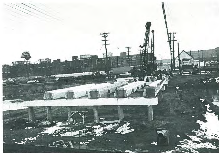
Fig. 24. Post-tensioned box girders on which pretensioned slab sections were placed. Topping was cast over the top of the deck section to provide a composite deck with girders and pretensioned slab sections.
