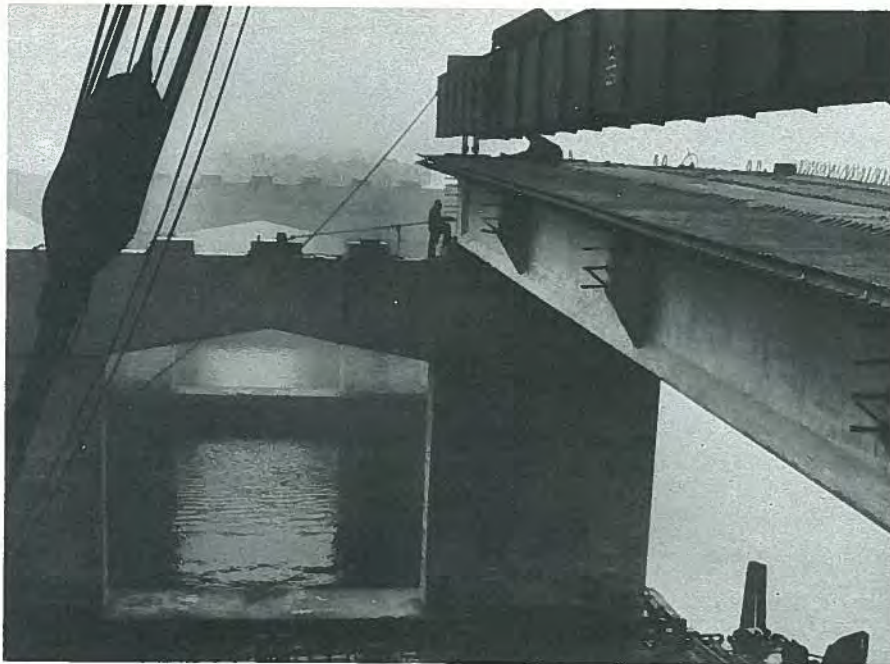
Fig. 8. Erection of 135-ft long precast prestressed concrete girders barged from Cape Charles, Virginia to Long Island, New York, a distance of about 350 miles, for the Cross Bay Boulevard Bridge Jamaica Bay, N.Y. Crossing. Owner, Triborough Bridge and Tunnel Authority.
