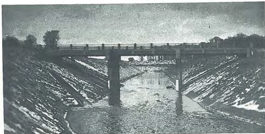
Fig. 10b. Completed three-span block-beam bridge in Tennessee.
