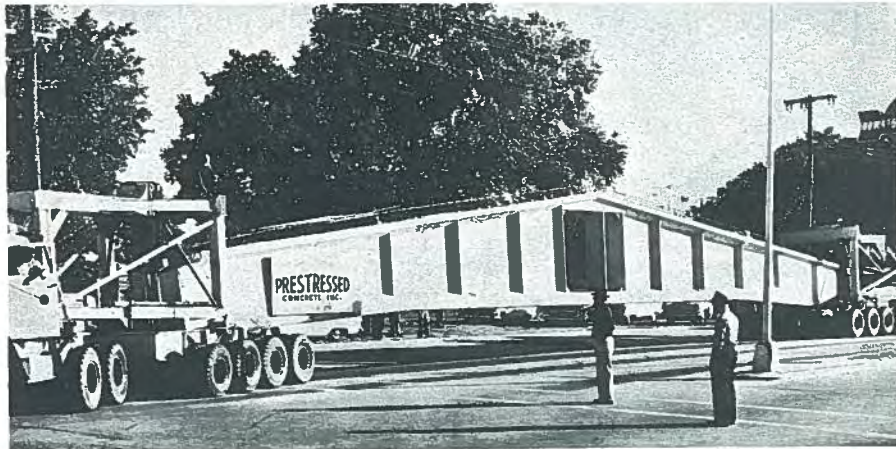
Fig. 5. Pretensioned tapered I-beam with opening and stiffening ribs being transported to American Cyanamid Corp's phosphate plant. Each beam was 101 ft (31 m) long and weighed 71 tons. Beams were fabricated by Prestressed Concrete Inc., in Lakeland (Courtesy, Paul Zia).
