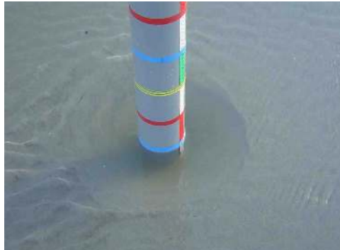
Figure 7.11 Scour around a test pile
